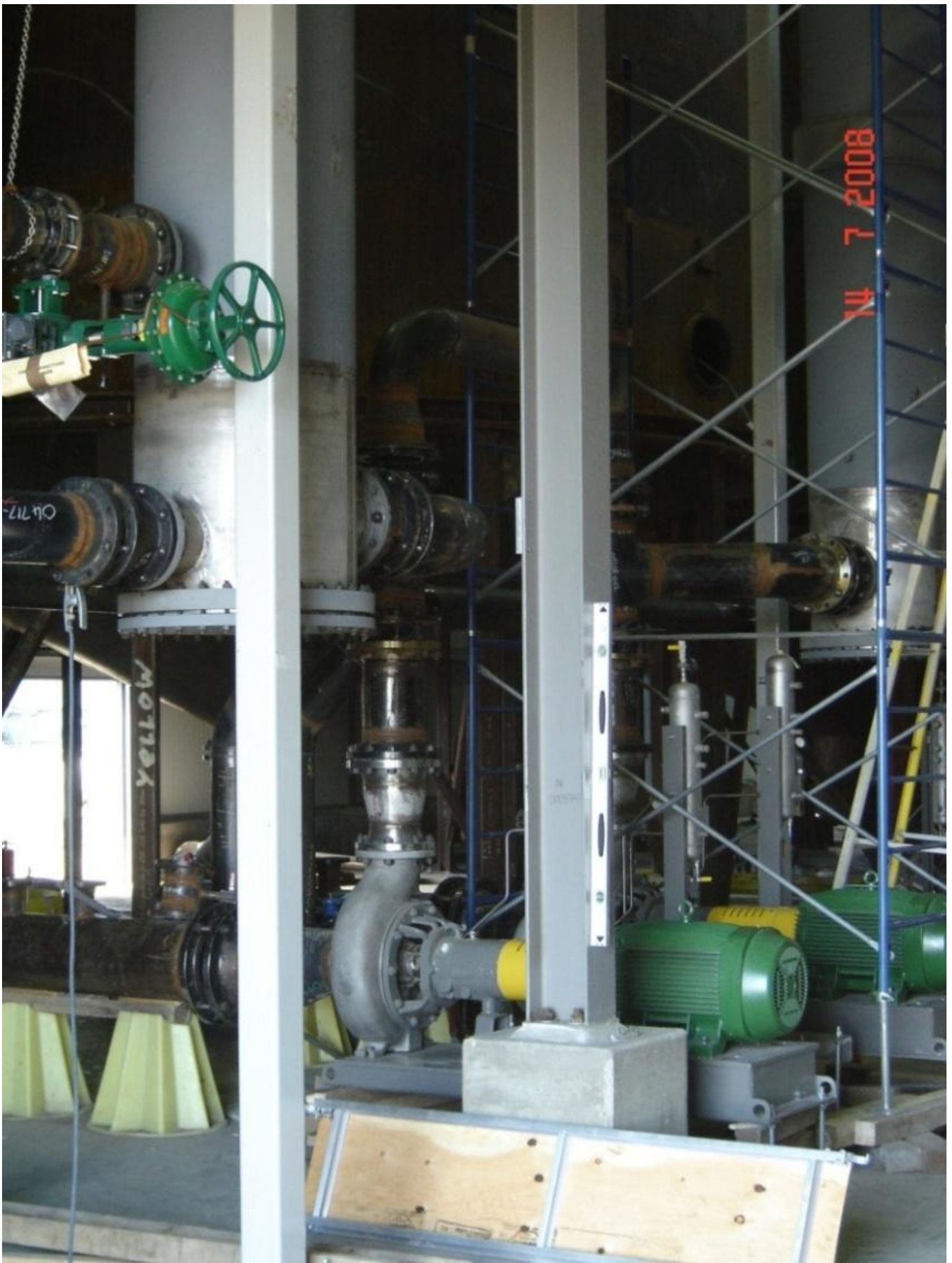
FERMINTATION PUMPS AND HEAT EXCHANGERS
